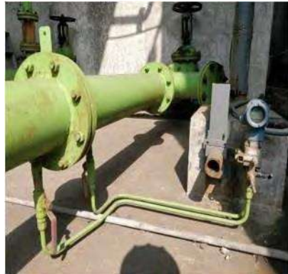
Water meter @inlet line
