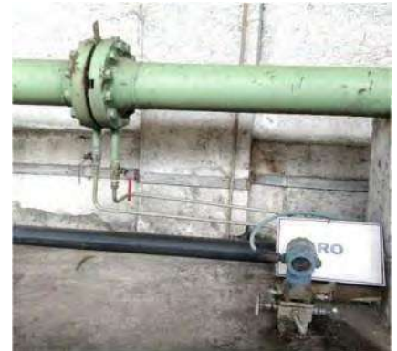
Water meter @reuse line
